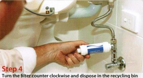
Simply reverse the procedure to replace the new filter
